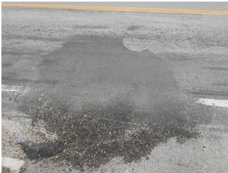
Figure 5.19 Patch Installed Using Infrared at Ohio SR 635
