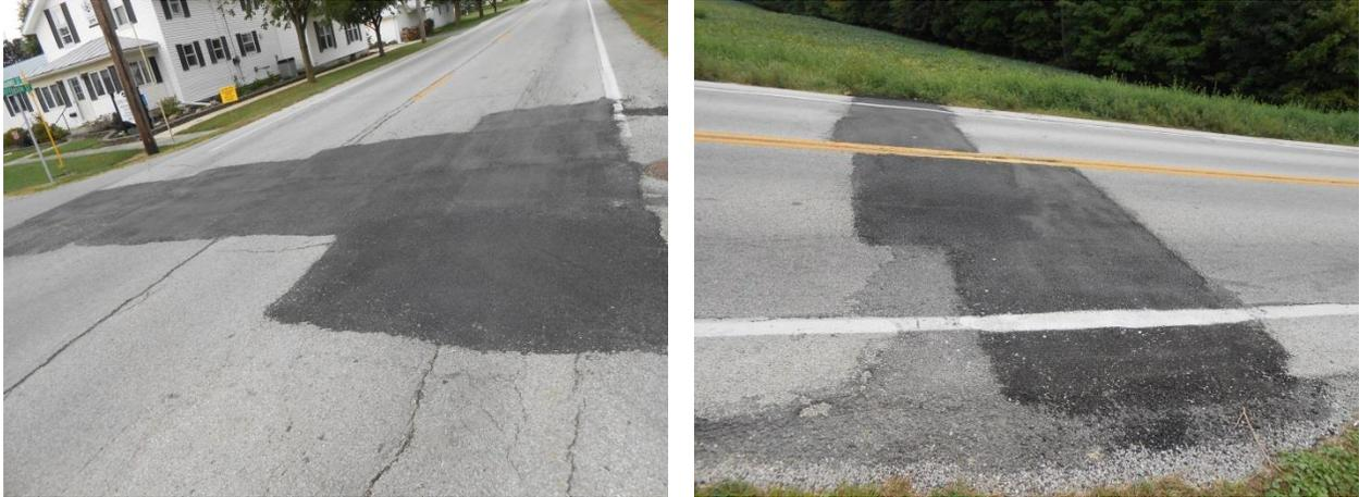
Figure 6.12 Infrared Patches installed on SR 18 after 30 Days of Installation
