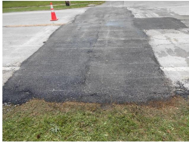
Figure 5.17 Infrared Patches installed at Ohio State Route 18
