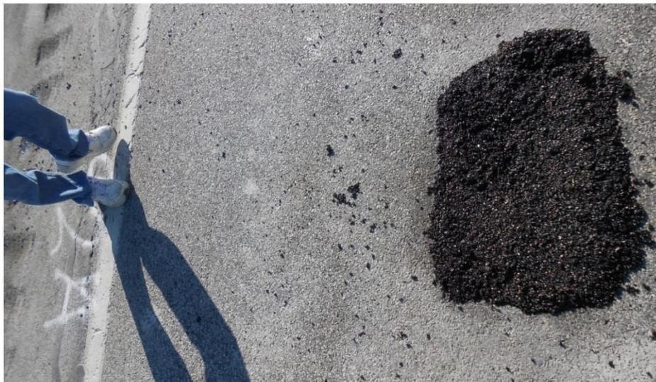
Figure 6.7 Right-After-Construction View Of A Throw And Roll Patch That Performed Well
