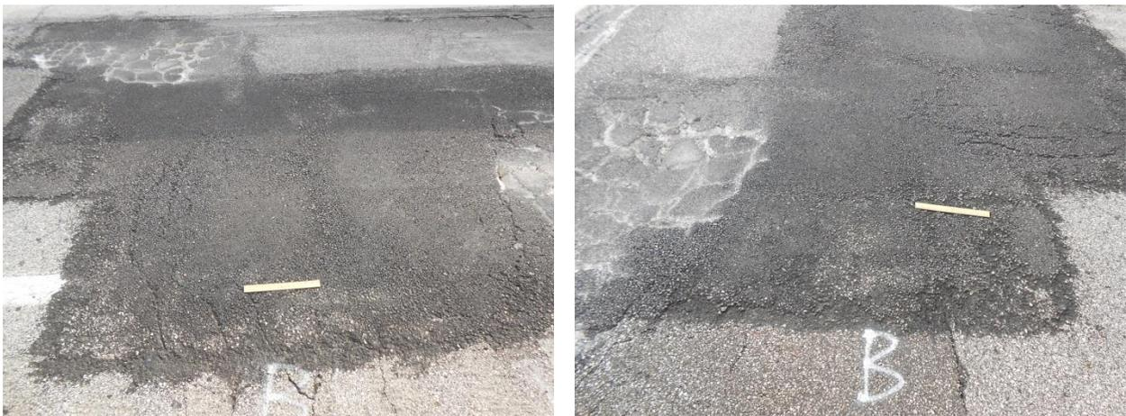
Figure 6.10 Infrared Patches on US 422 after 70 Days of Installation
