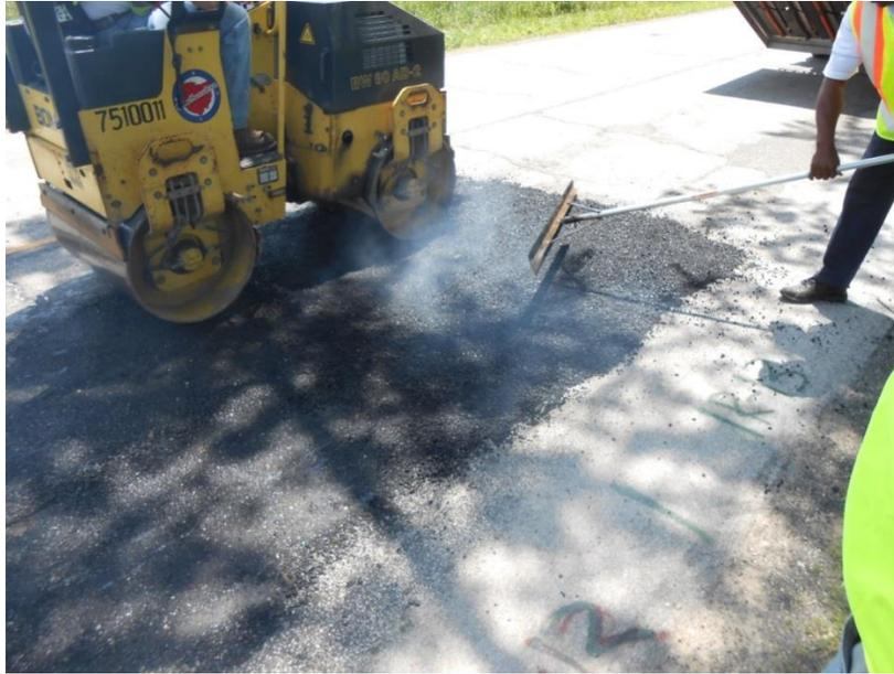
Figure 5.13 Patches Installed Using Infrared Method 3 at SR 168
