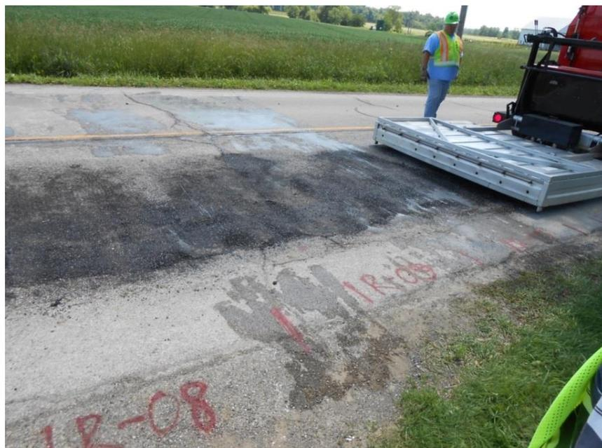
Figure 5.12 Patches Installed Using Infrared Method 2 at SR 168
