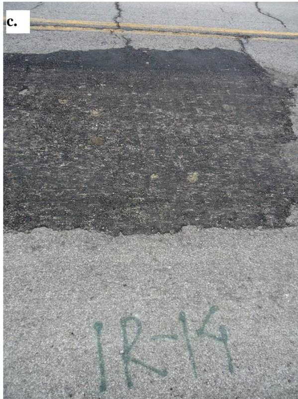
Figure 6.11 Infrared Patches installed on SR 167 after 30 Days of Installation
