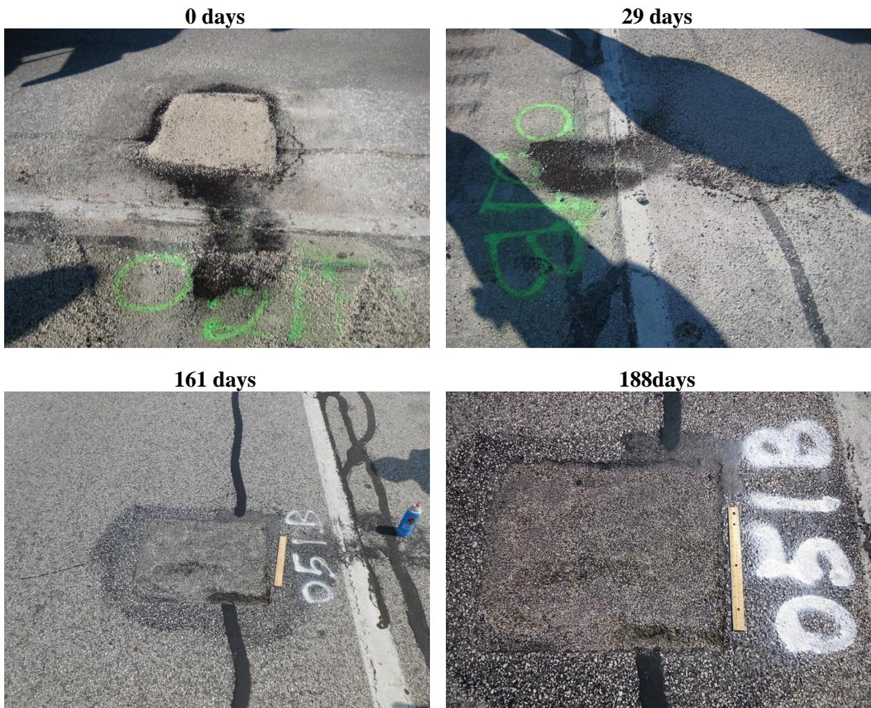
Figure 6.5 Pictures for a Spray Injection Patch after 0, 29, 161, And 188 Days Of Installation
