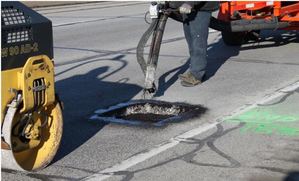
Figure 5.6 A Picture Taken During Patching A Pothole At I-480 Using Spray Injection Method
