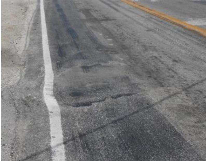
Figure 5.18 Distressed Pavement Area That Was Patched at Ohio SR 635
